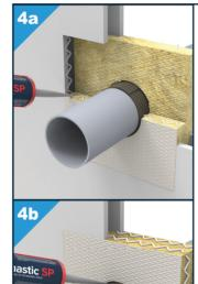
Close the remaining gap according to the Multimastic C System or Multimortar System.
